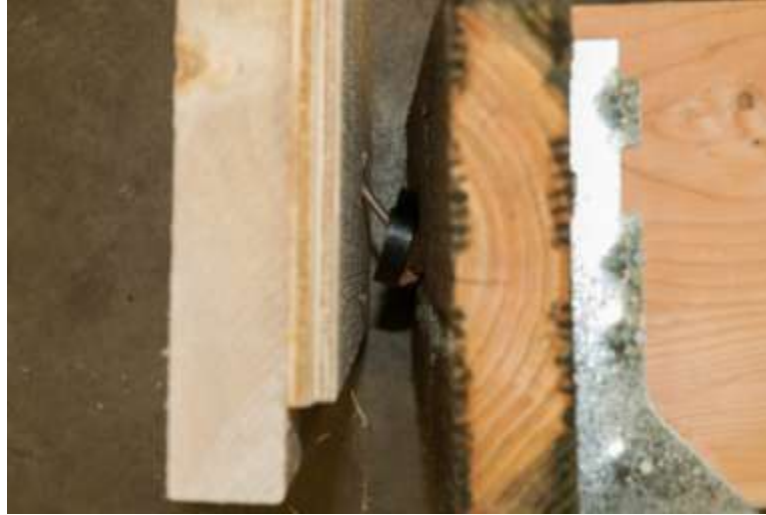
Figure B17. Typical Failure for Configuration 5, Simpson SST Ledger Screw
